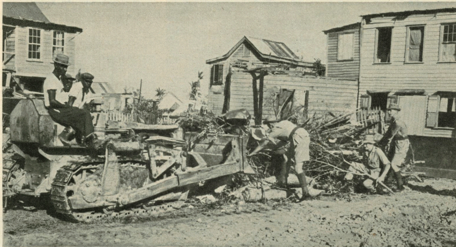
Bulldozers and heavy equipment brought in by the Plant Section of 12 Field Squadron were used to clear away the piles of debris.
