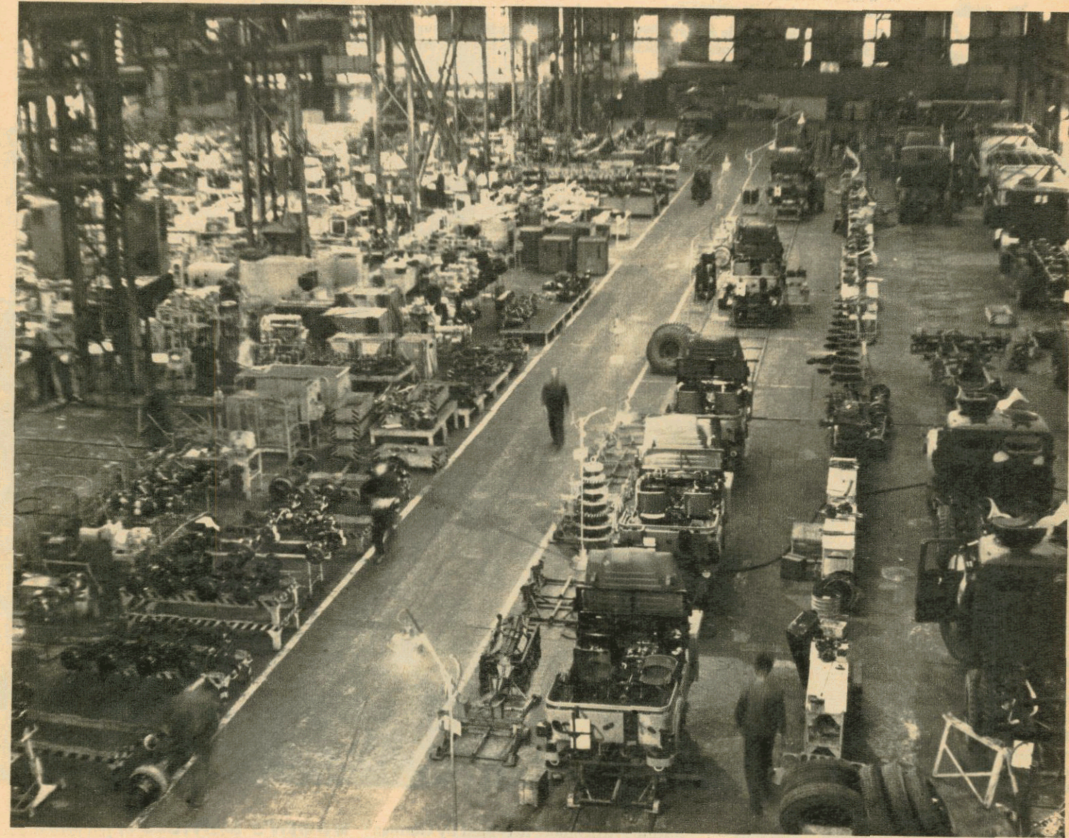
A bird's-eye view of 23 Base Workshop's gigantic shed where soft-skinned vehicles are dismantled, tested and made fit for the road again.
