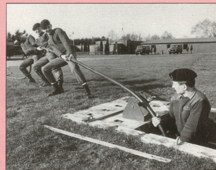
Signallers remove old cable from a communications duct at RAF Bruggen. All part of their work in support of the Royal Air Force
