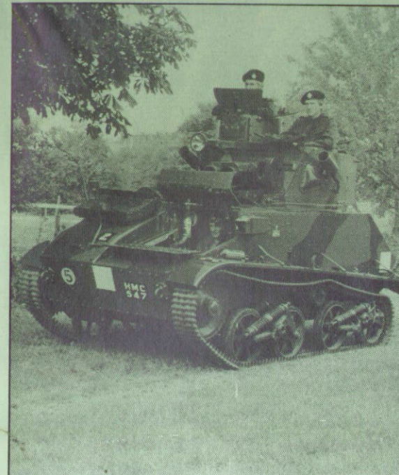
The 1938 model Light Tank Mark VIB. It carried a crew of three and mounted two machine guns in the recce role.
