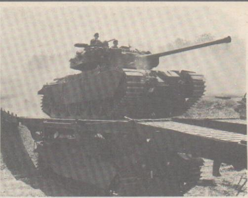
The new *Ark* bridge-layer in action. It simply drives into the gap to be crossed and, opening out its tracks, forms a safe, stable bridge.
