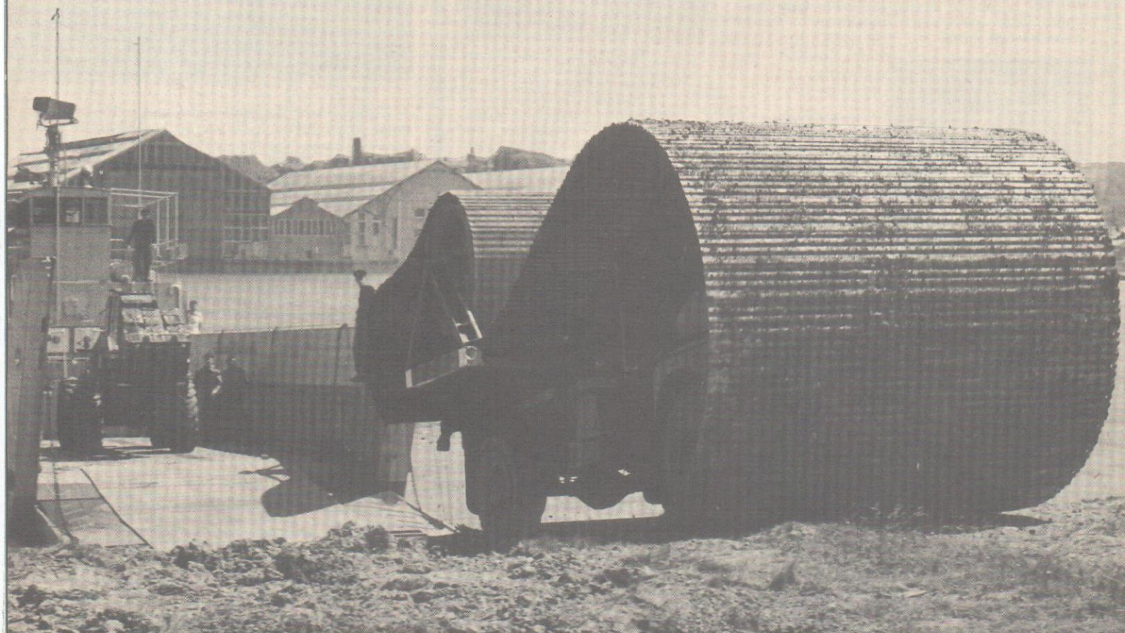
Landing on the banks of the River Medway, the lorry-with-a-built-in-road has no trouble crossing the mud, and leaves the track for following vehicles.
