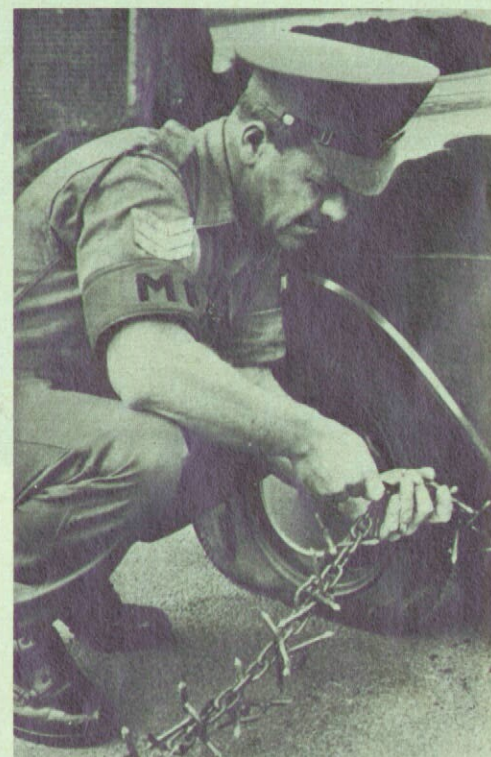
An ancient device comes to the aid of troops in Northern Ireland. The caltrop, which always lands with the spikes sticking upwards, was used by the ancient Greeks against cavalry. More recently it has been adopted by the Viet Cong. Its use in Northern Ireland could stop cars driving through road blocks.
