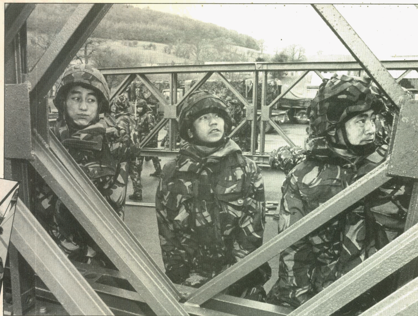
Gurkhas of 69 Gurkha Fd Sqn take the strain as they construct a medium girder bridge
