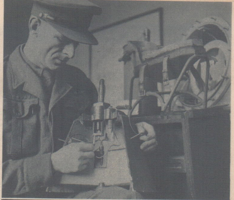
The SME's mines expert, Capt. J. P. Ewart (left) is showing the way a single-horn Japanese beach-mine works. Just above it is a mine-shoe, which will stop a Schu-mine from blowing off your foot, though it will still shake you.
