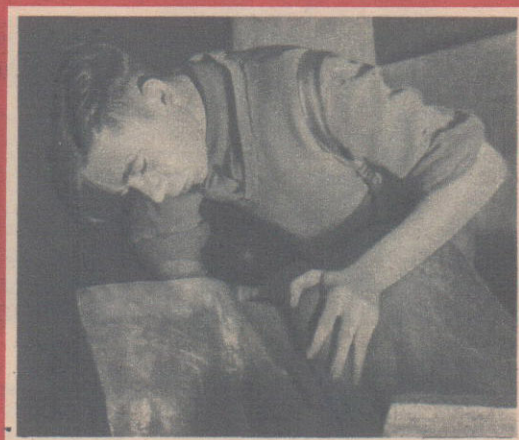
Beating a sheet of lead into corner guttering for a roof is this Sapper's trade-test.
