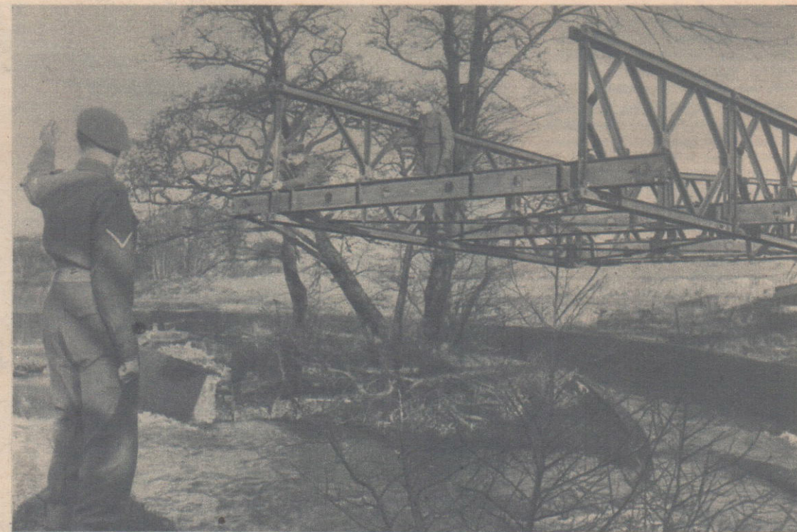
Creeping across the Ure is a Mobile Bailey bridge, built in sections on rubber-tyred wheels and towed to its site.
