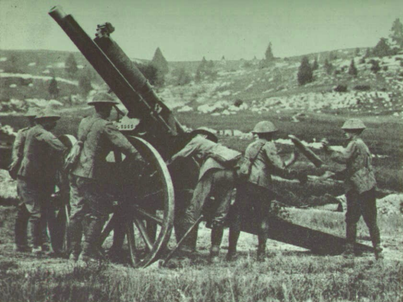
Italian front, World War One—18-pounder on special anti-aircraft mounting.
