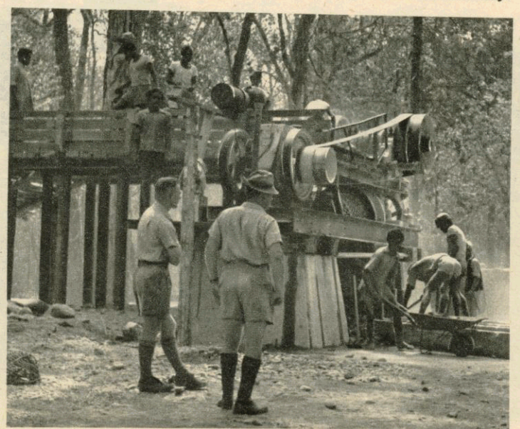
Below: S/Sgt. J. A. Heard and Sgt. R. H. Baker supervise the grading of stones for road maintenance. River-bed boulders keep the stone-crusher busy.
