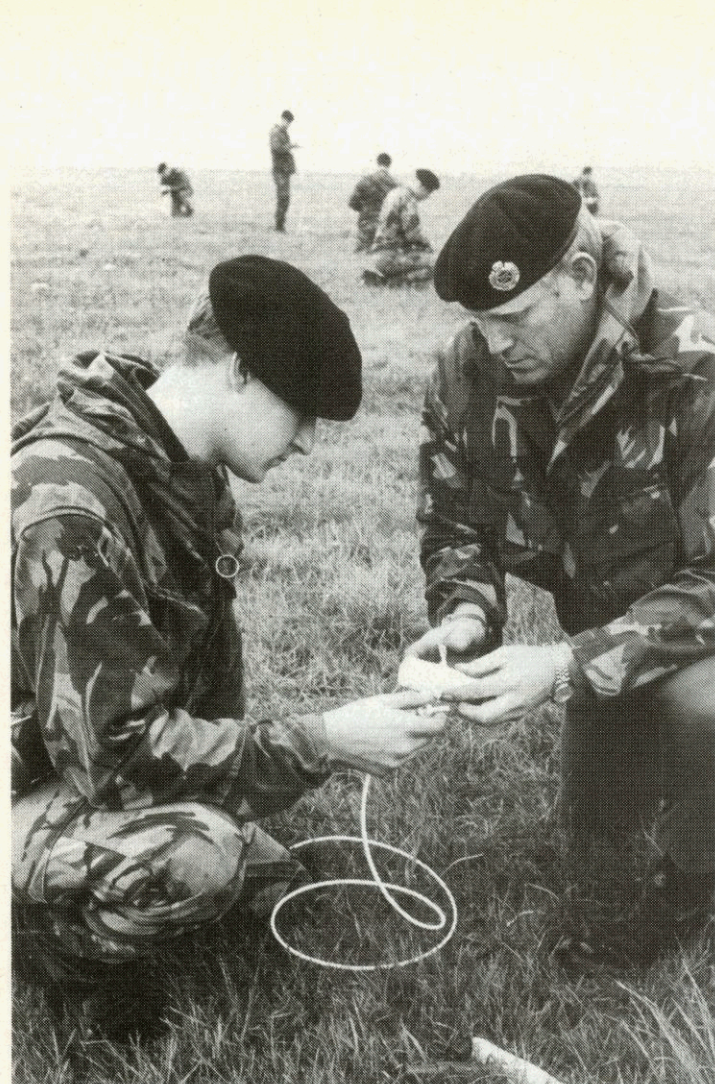
Above – QMSI Ken Mason RE (right) shows Tpr Darrell Fordyce how to set up a demolition charge
