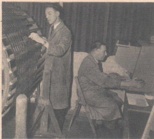
At the micro-film camera: the operator in this picture is photographing soldiers' records of service. The actual camera is above the operator's head. Below: On the left a film is drying. On the right is the "reader" on which films are checked before they are sent off.
