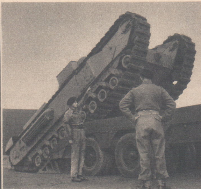
Up she goes! A trainee at Ranby Camp, Notts, rehearses loading signals to guide the driver of a tank transporter as he operates the tractor's winch.
