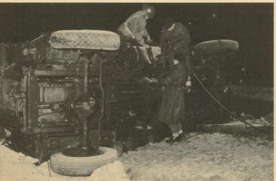
*Scammell* positioned on firm ground, anchored with a gun plank driven into the earth between its rear wheels.
