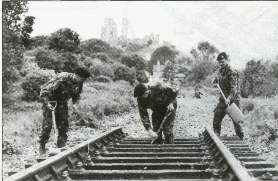
Members of Manchester-based 75 Engineer Regiment (Volunteers) RE relay 400 yards of the Purbeck Line track into Corfe Castle station, Dorset. The 24-hour operation by the TA sappers was part of their two week camp and gave them a unique opportunity to build from scratch a railway line which will be put to regular use
