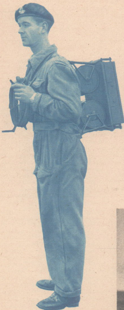
Above: Corporal W. Melville, stationed on Hohne Ranges, shows how the Hohne Box, weighing 30 pounds, can be carried on a man's back. Right: By pulling a wire (which can be as long as desired) the magic box can be made to set off distant explosions.
