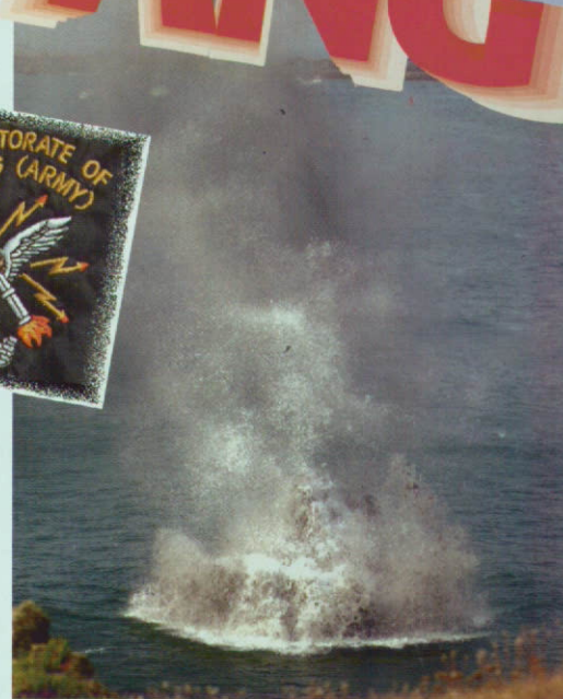
Making waves: RE divers use explosive to shatter a massive rock obstructing anchorages in historic Alderney Harbour
