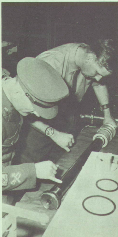
Above: Warrant Officer Jim Ware inspects damage caused by dirt to a piston. Right: Technicians in white rubber boots at work in the Clean Room.
