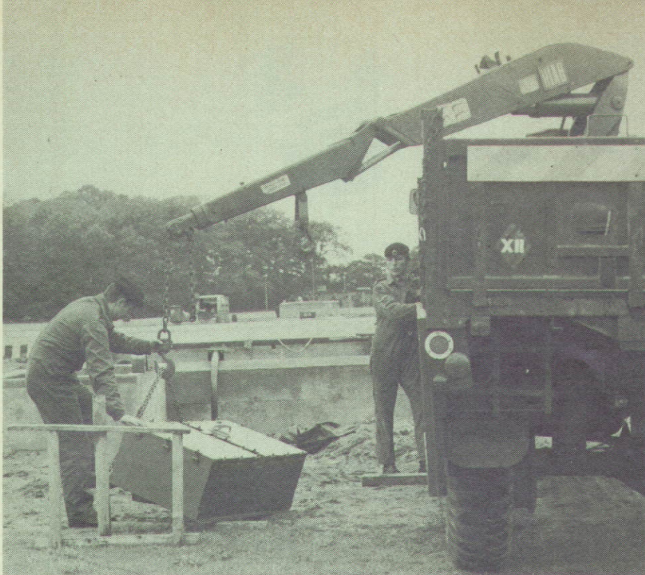
Left: At Leuchars the control box of the arresting gear is lifted into place.
