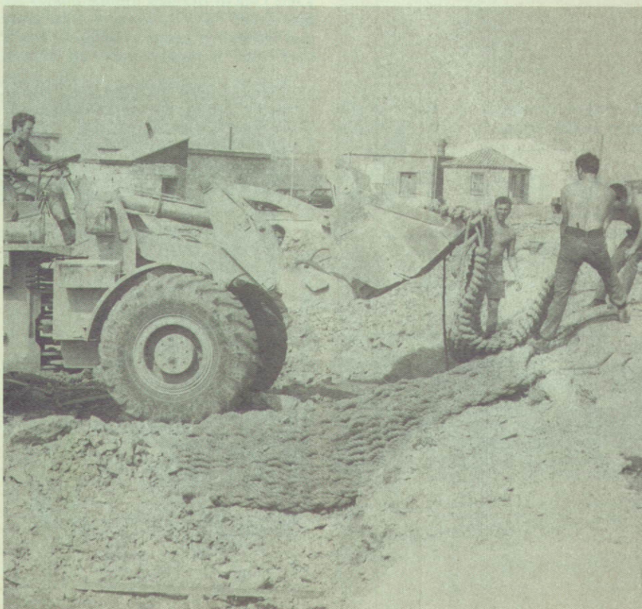
Left: Rock blasting is about to start at the Europa sports pitch. Thick rope nets stop damage to nearby houses.
