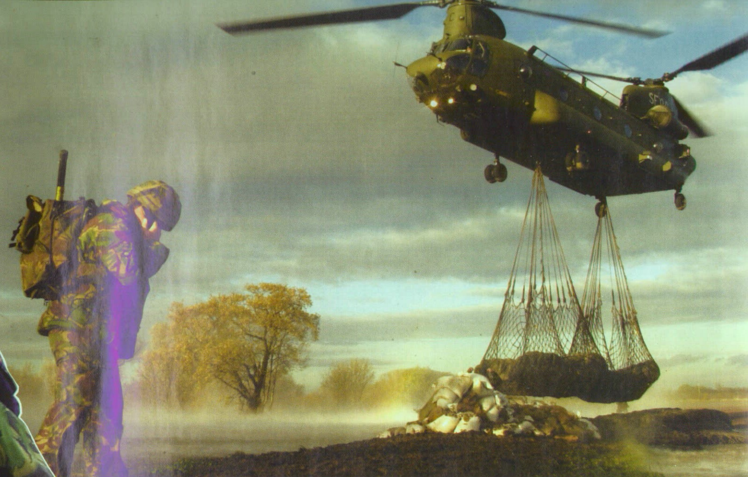
Plugging the hole: RAF Chinooks drop blocks, made from recycled tyres and delivered by 10 Tpt Regt, into a breach in flood defences near Howden
