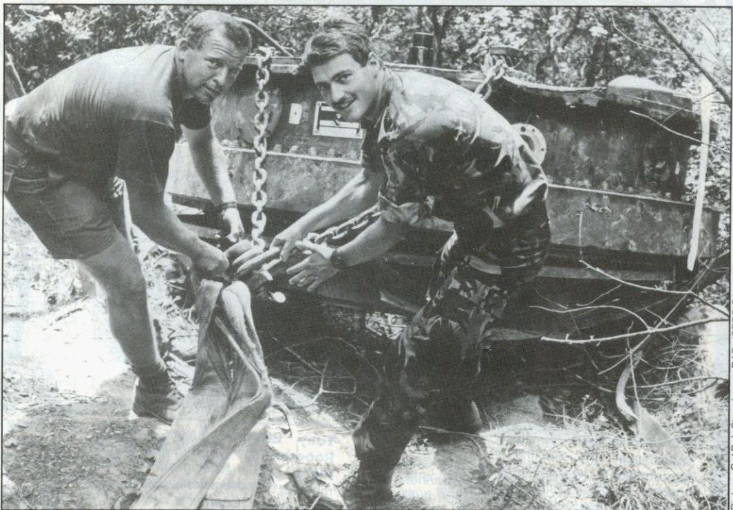
The start of a busy afternoon for Sgt Frank Taylor (left) and Capt Phil Ingram as they check securing shackles on the radar turntable before the winching operation began
