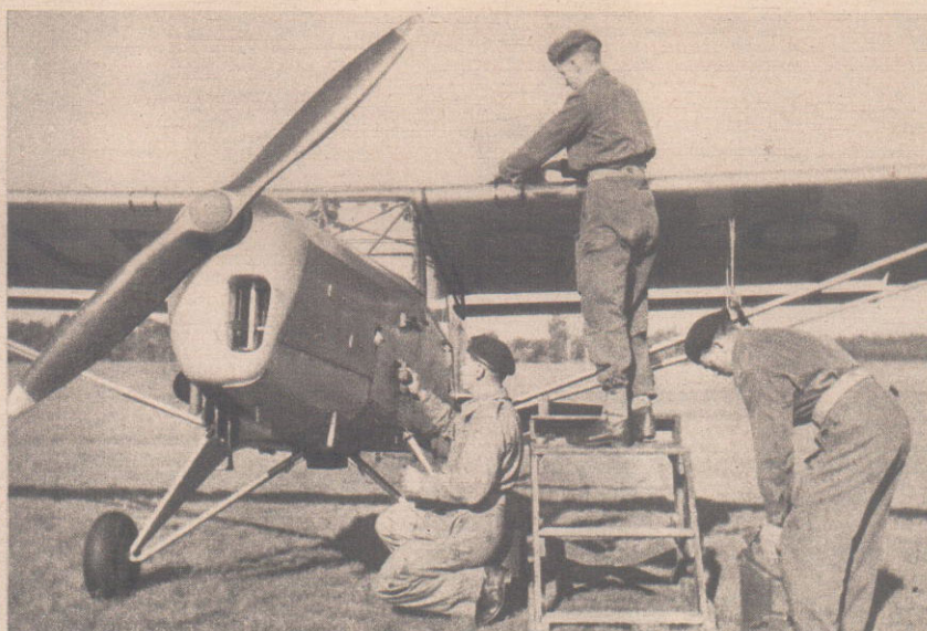
Left: In stormy weather an Auster must be tethered to the ground. Here students learn how to set out pickets.
