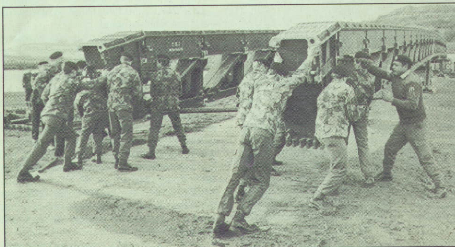
Below: Assembling double span girder bridge.
