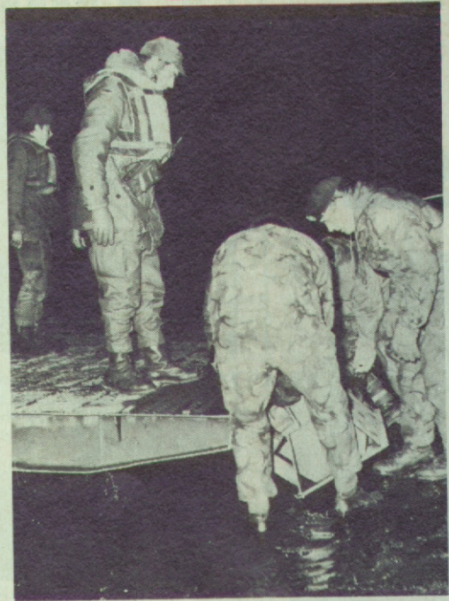
British and German sappers combined to build one of the largest M2 units ever constructed in Germany in just over two hours over the 400-metre-wide River Elbe. The bridging was the finale to a week's training by the British 28 Amphibious Engineer Regiment and a company from the Amphibisches Pionierbataillon 130 of the Bundeswehr. The two units both use the German-designed bridge, which can double as a ferry.
