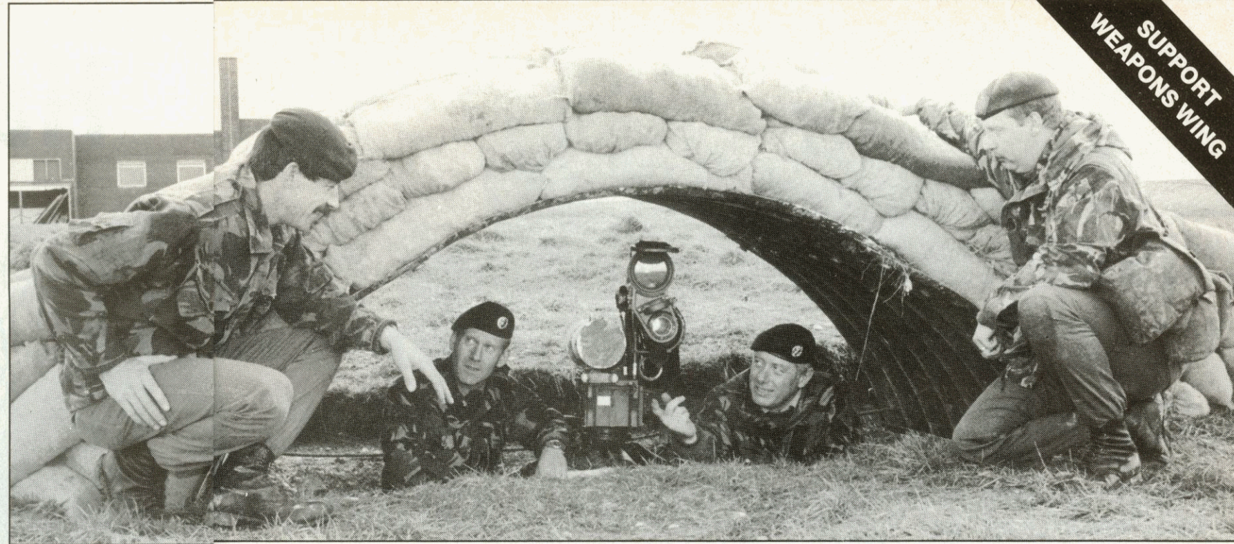
Above right - Typical SWW instructors show SOLDIER the Chatham Arch - originally sapper equipment intended for building culverts which can bear heavy loads. It is
