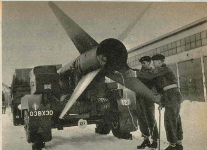
Above: Here the fins are fitted and the five-ton Honest John is ready to be towed away to its launcher.
