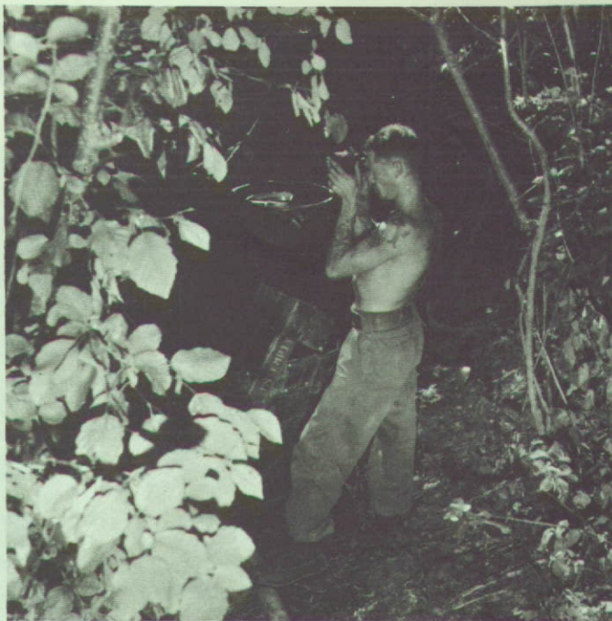
Water is a Service Battalion responsibility. An engineer tests water in a camouflaged treatment unit for purity.
