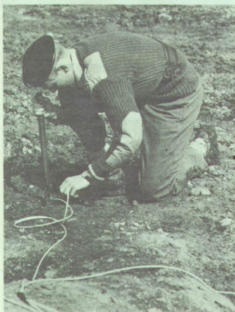
Rocks that dotted the proposed airstrip had to be got rid of. Top: Preparation for blasting.
