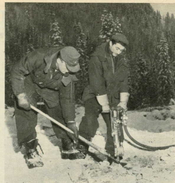
Spr H. W. Hawes (left) and Cpl D. E. Reeves drilling a hole for a dynamite charge to level an approach to the bridge. Below: Spr L. F. Wollshlager, Spr J. P. C. Morettin and L/Cpl J. D. Howie busy laying planking.
