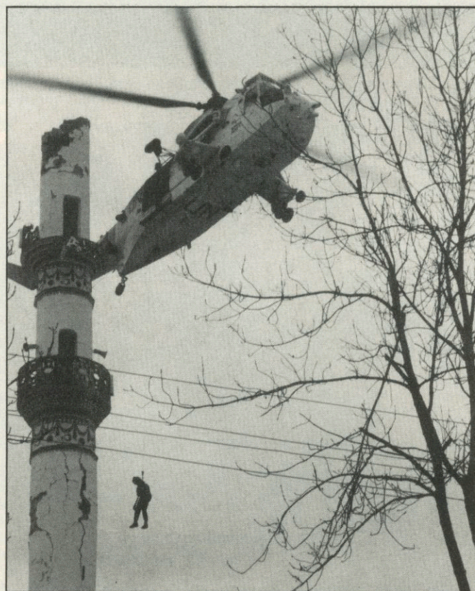
Sappers, with the help of a Royal Navy Sea King helicopter, prepare to topple a war-damaged minaret tottering over a village
