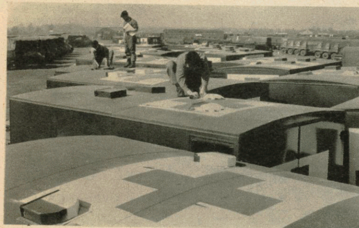
In the battle against the Battalion's bitterest enemy—the weather—a maintenance team seals up ambulances to make them 100 per cent waterproof.
