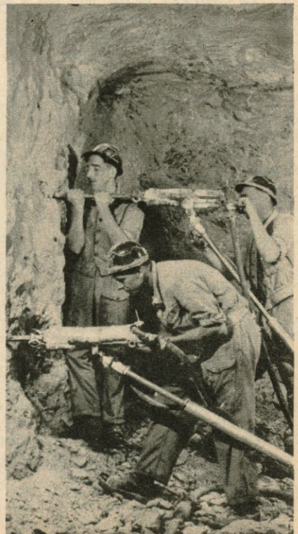
Right: At the tunnel face the explosives are plugged into holes made by these compressed air drills. Sapper Danson steadies the bit as Sapper Bullivant withdraws the drill, while Sapper Harrison makes a new hole.
