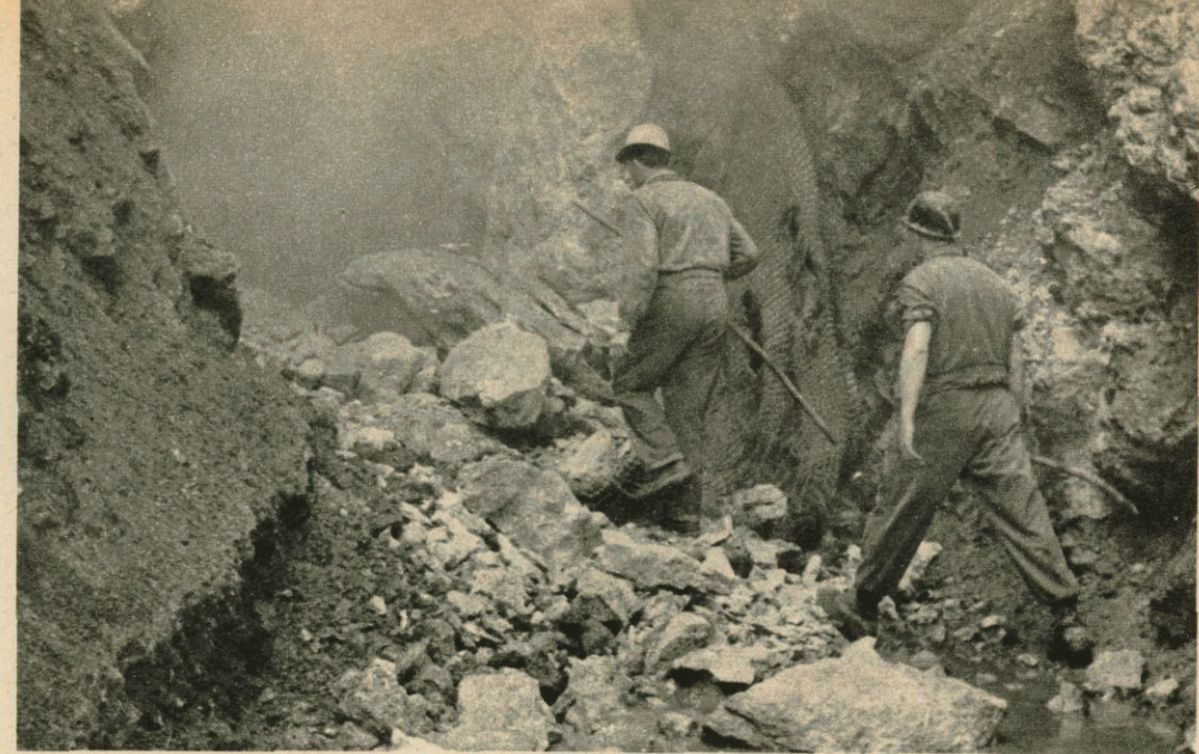
Wearing miners' helmets, Cpl Stones and Cpl Dunn, of the Tunnelling Troop, pick their way into the smoke-filled tunnel over debris brought down by shot-firing. Their job is to inspect the roof after the final break-through of Harley Street, the latest triumph.
