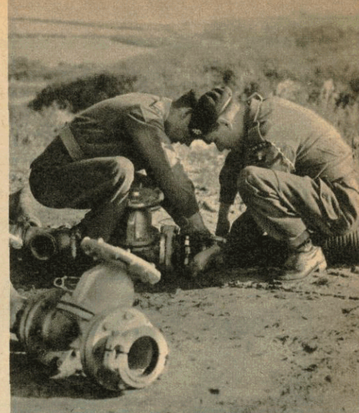
Right: Linking up the flexible pipe which carries the fuel from the sea to storage tanks. Damaged pipelines can quickly be repaired.
