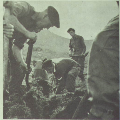
Above: Digging out to make a level bed for the cable after explosives had done the heavy work. Below: The cable will be difficult to repair, so junctions were very carefully sealed with pitch.
