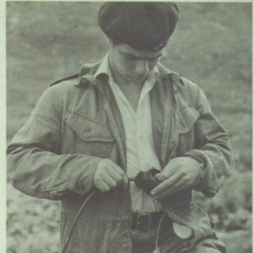
Above: Digging out to make a level bed for the cable after explosives had done the heavy work. Below: The cable will be difficult to repair, so junctions were very carefully sealed with pitch.
