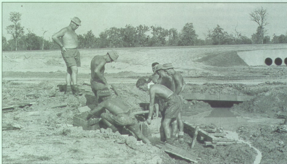
Draining work: This Soldier photograph from June, 1965 shows men building a culvert at the Loeng Nok-Tha airstrip site. Drainage was a big challenge during Op Crown (see below)
