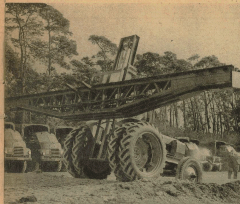
Build your Bailey bridge this way: the fork-lift truck carries two steel bridge girders like these to the scene of operations with ease
