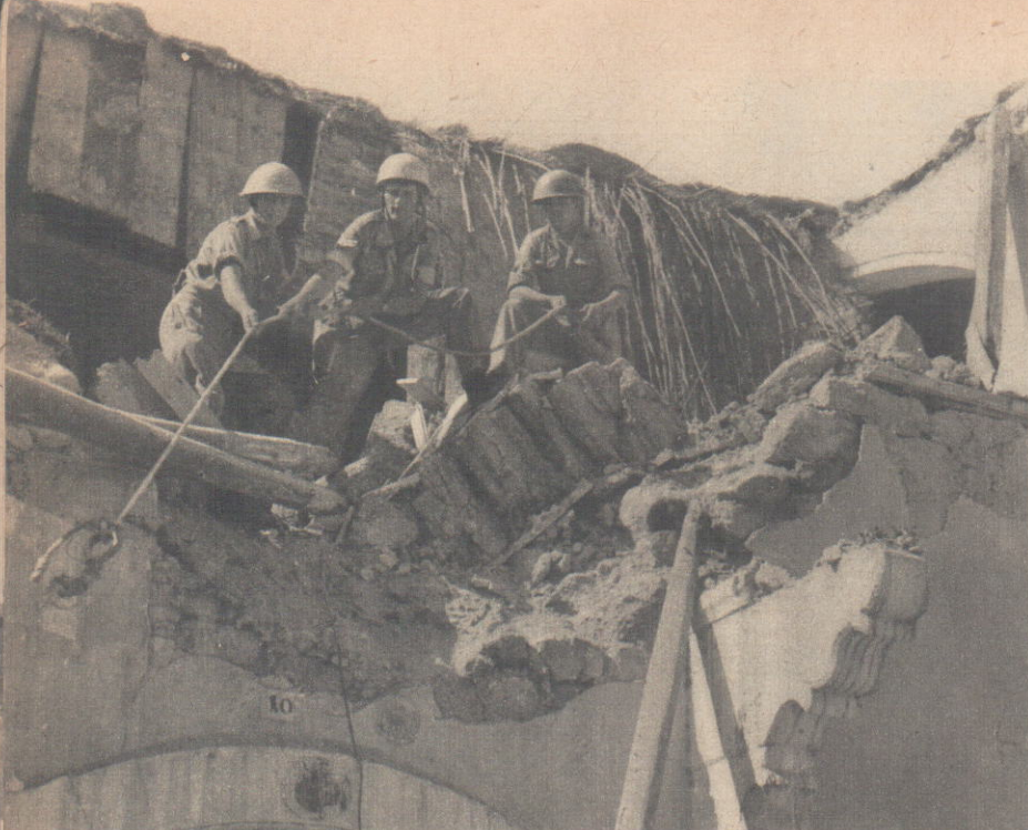
The earthquake started it—the Army finishes it. Tottering walls cannot be cleared by explosive; they must be pulled down. Here Sappers set their gear.
