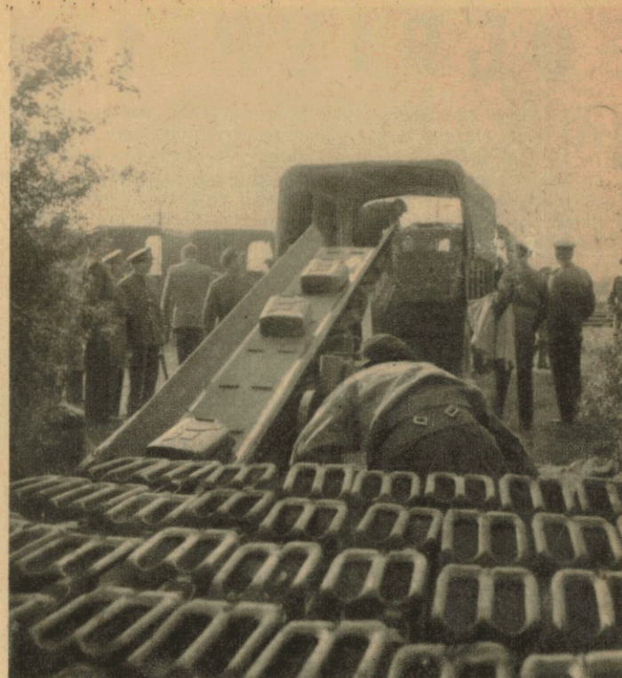
This transporter runs on a single rail and requires no driver. It may soon be used in big depots. Right: the new conveyor belt loading petrol cans.
