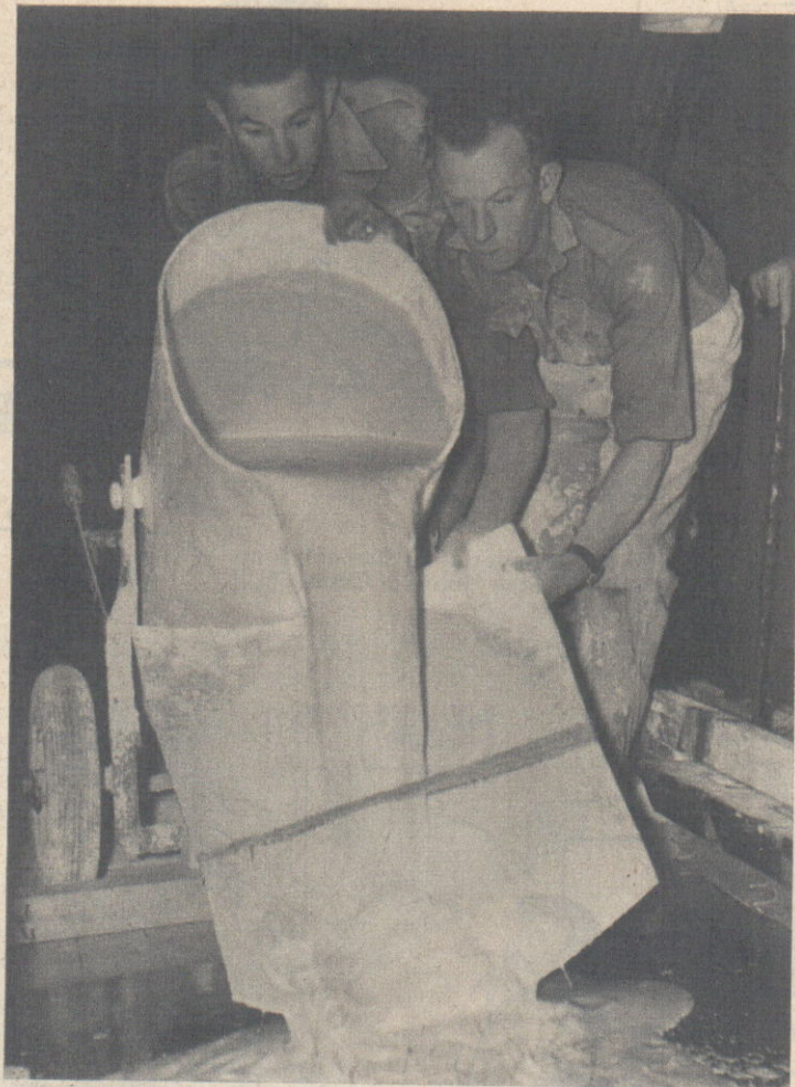
Here's a wall being poured out while you watch. In 20 minutes the gypsum plaster will have solidified in its mould. Below: the wall is hoisted into position.
