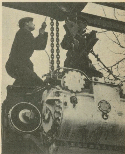
The school trains tank mechanics as well as Cavalry and Bersaglieri. Here, trainees are instructed in tank engine maintenance.
