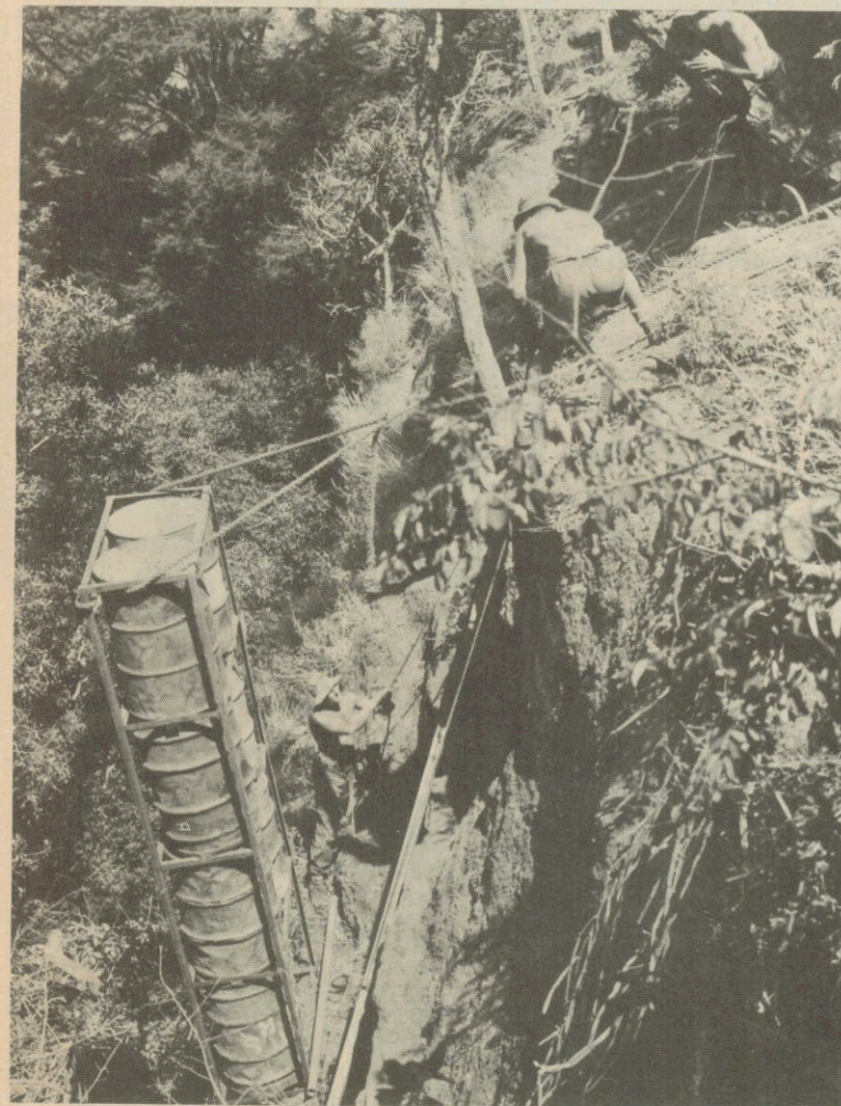
Men of 34 Independent Field Squadron, Royal Engineers, lower a section of a prefabricated raft down to the water.
