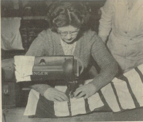
This membrane being sewn into the sleeping bag forms deep pockets for the down and ensures warmth.
