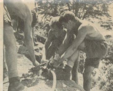
Drilling holes for plastic explosive charges.
