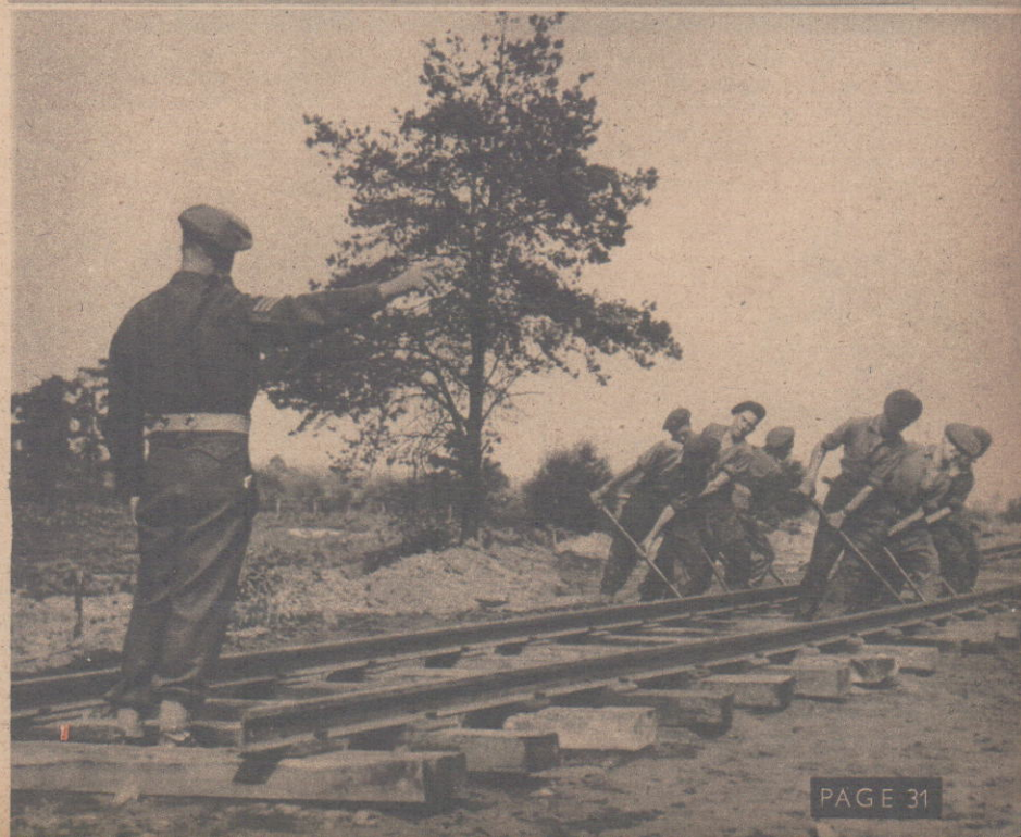
The Ross fork lift will heave loads up to 6½ tons on working days; at the Longmoor "At Home" it carried up to 20 children both up and down and backwards and forwards. Below: How to man-handle a railway track. If you don't like your railway's route, just get a gang of men and some crowbars and shift it somewhere else.
