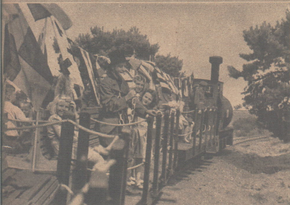
Stephenson might have been proud of this one. Its smoke-stack wobbled on springs and the floors of the wagons pivoted on bends. But the power was provided by an up-to-date diesel locomotive in fancy dress.
