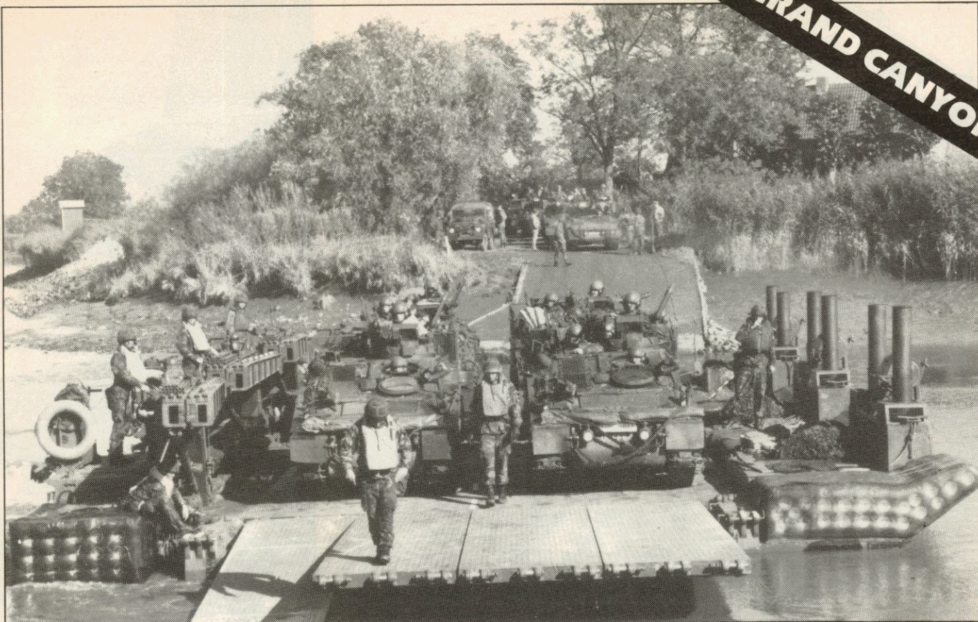
M2s of 23 Amphibious Engineer Squadron ferry Spartans of the 16th/5th The Queen's Royal Lancers across the River Jumme. The M2 is a 22 ton amphibious military vehicle designed for use on water as a single ferry. It can be linked to other M2s to form a larger ferry, or to make a bridge across a river. As a vehicle it can be driven on highways or cross country
