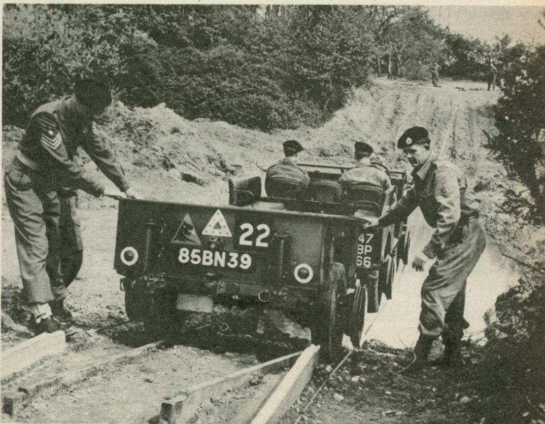
Sappers carefully check that the cable fits into the hubs as the Land-Rover and trailer leaves the guide and begins its 200-ft journey. The bridge and its equipment is carried in two Land-Rover trailers.
