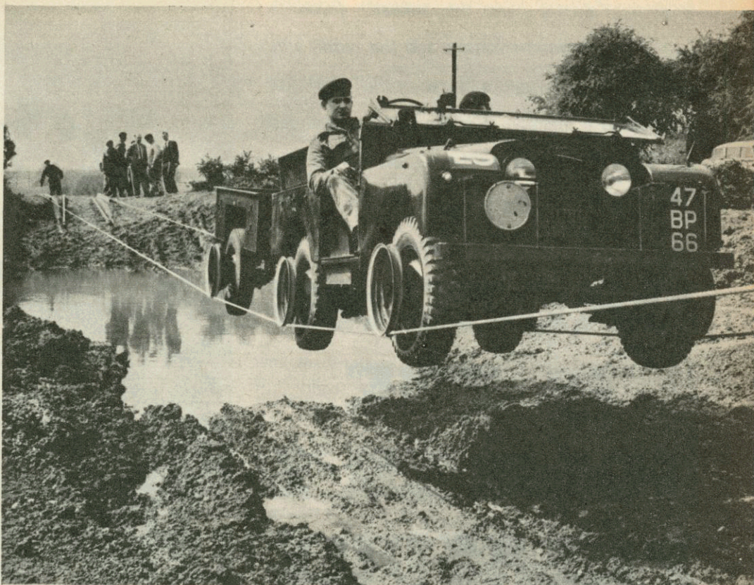
The steel cable sags only slightly as Cfn D. Chapman, REME, drives his Land-Rover and trailer over the Miller Bridge. The hubs on which the vehicle rides take only a few minutes to fit. Similar bridges, erected to the required width, could also be used for passing over most of the Army's light vehicles.
