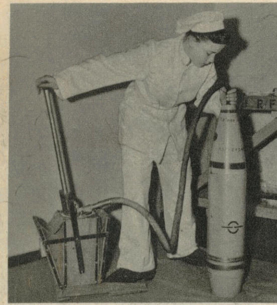
With a hand-operated vacuum cleaner, Private Cowley extracts fragments of a broken exploder. Note the protective uniform.
