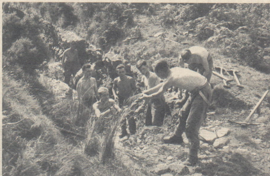
A retaining wall of sandbags replaces the bank washed away by the river Exe at Dulverton.
