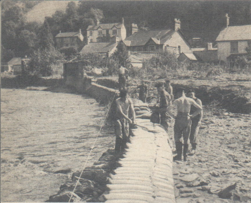
A retaining wall of sandbags replaces the bank washed away by the river Exe at Dulverton.
