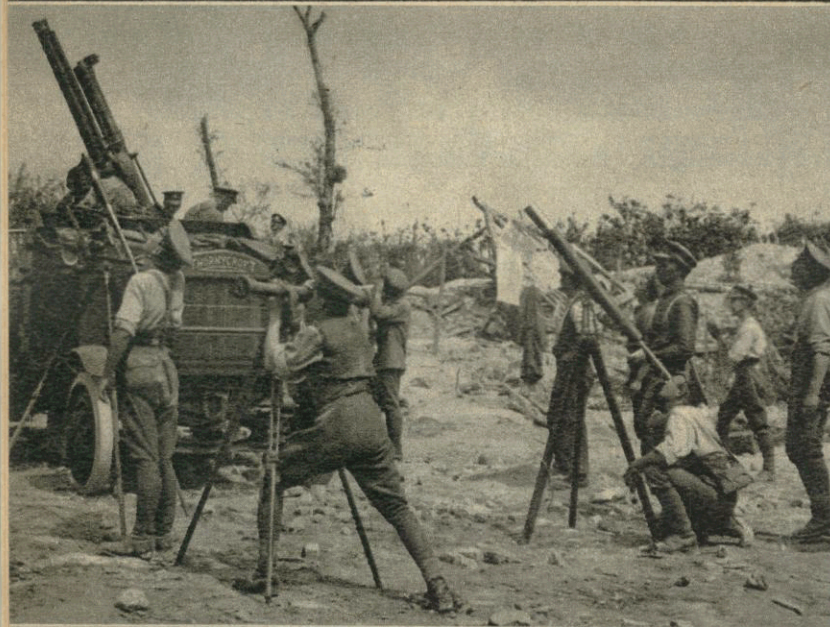
Fricourt, France, August 1916: a 13-pounder anti-aircraft gun mounted on a lorry goes into action. Tripod-mounted telescopes are used for spotting. A range-finder is being operated by the soldier in foreground.
