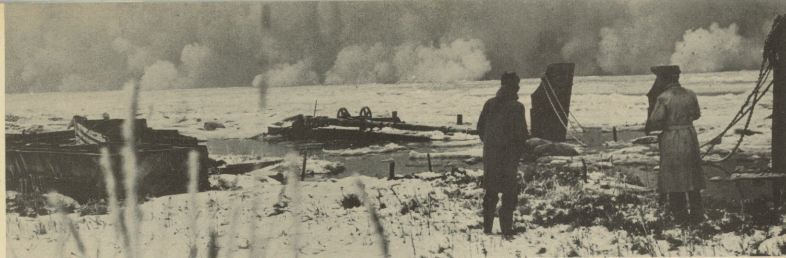
Working in a race against the rising tide, a small party of Sappers gingerly laid charges on an ice-choked river at Colchester in Essex. The men, from 36 Corps Engineer Regiment at Maidstone, had answered an urgent call from the town to clear the river so that four stranded ships could be freed and barges bringing urgently needed coal could unload their cargoes. Using plastic explosive, the Sappers opened the river by exploding the ice—up to ten inches thick in places—with more than 70 charges laid five yards apart along the river. And they completed the job only just in time. Tide rising over the ice threatened to trap the Sappers in mid-river—the last man had to be hauled to safety.
