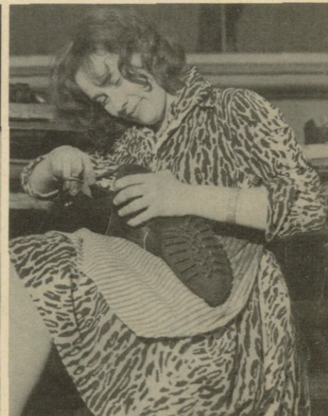
Beauty and the boot? After welding the rubber sole is trimmed by hand.
