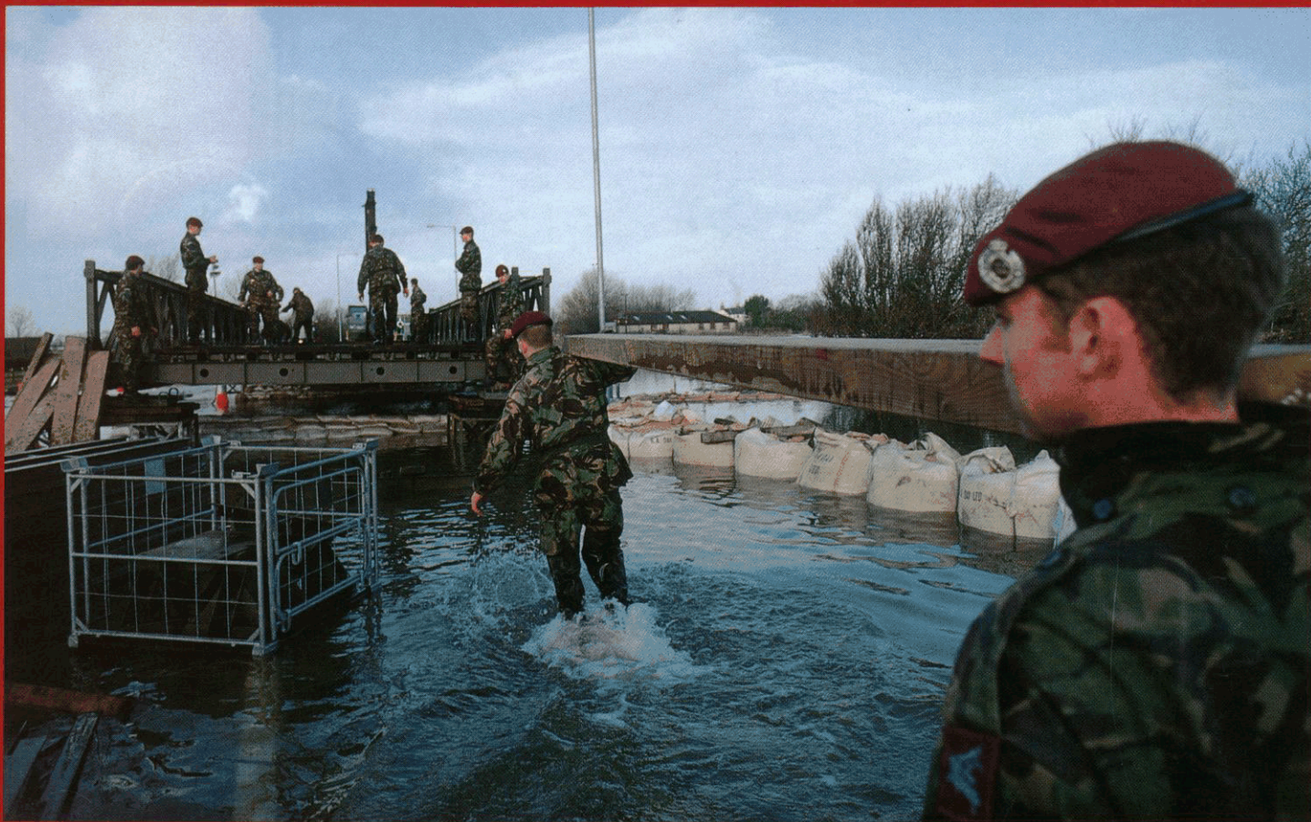
Sappers of 9 Parachute Squadron RE waded through flood waters in the West Sussex city of Chichester during Operation Aquaplane. They and other Army engineers built Bailey bridges across flooded roads and filled thousands of sandbags in the fight to hold back the deluge. Full story in Pages 14–15.
