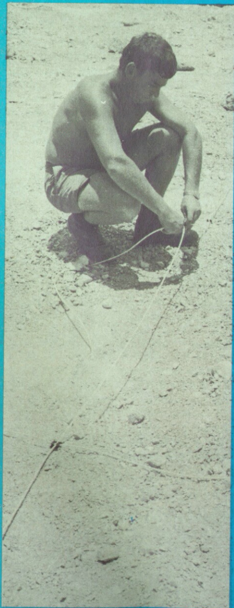
Below: Charging lead check before blasting.
