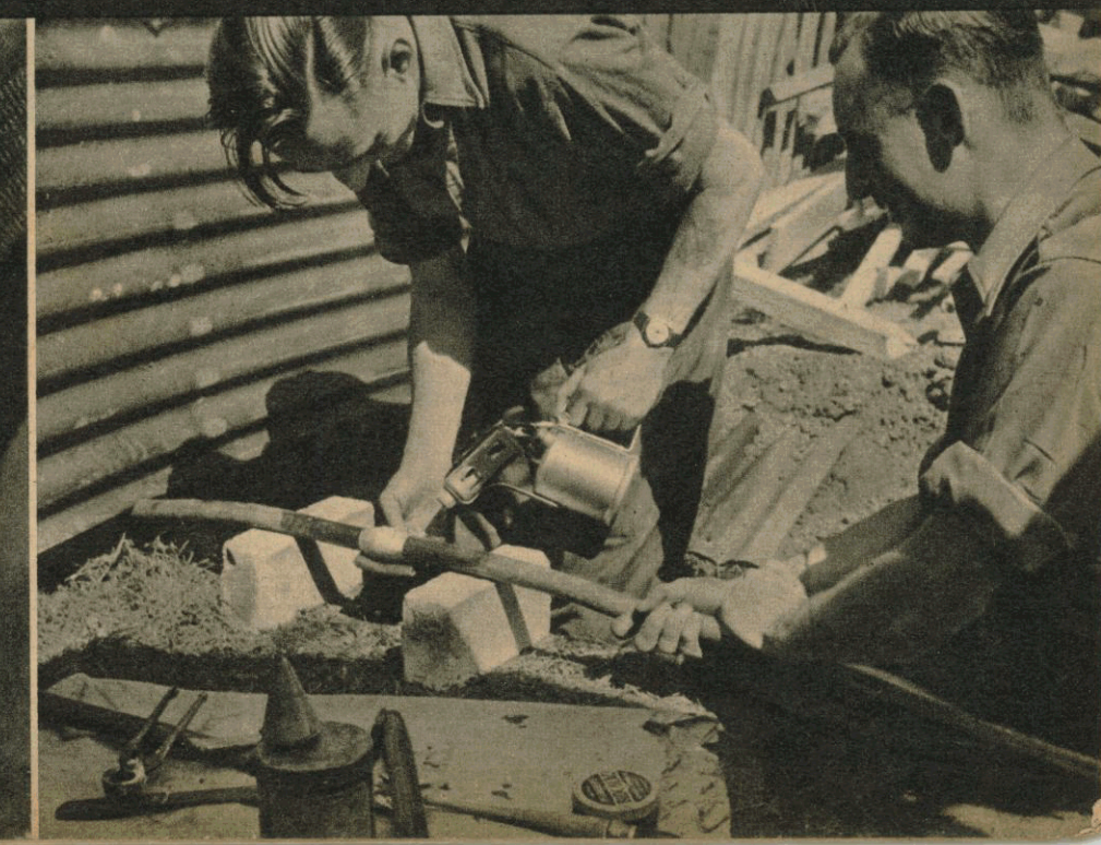
The soldier-builders are divided into seven groups, each doing a separate job. Above, bricklayers are seen learning to mix cement, and below a professional-looking joint is being made in a lead pipe by a learner under his instructor's guidance.
