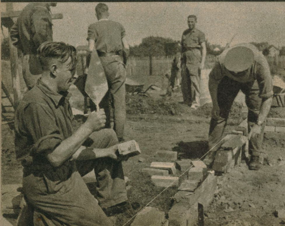
Below: The first courses of brickwork being laid. The builders work in pairs, an expert and a learner.
