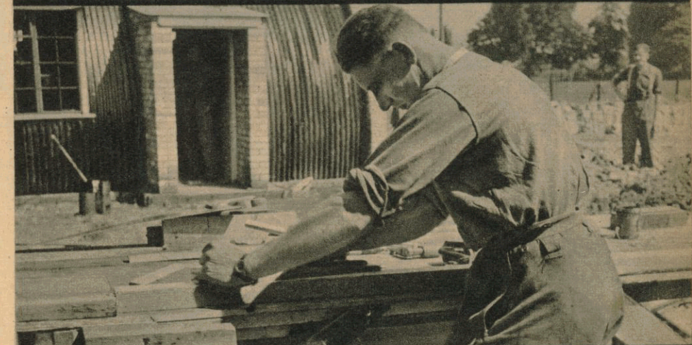
Timber, obtained from salvage, needs much planing and reshaping before it can be used, but it's all good practice.
