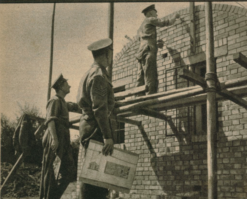
Above: An end wall goes up. It is neat and workmanlike. No jerry-building for the Guards.
