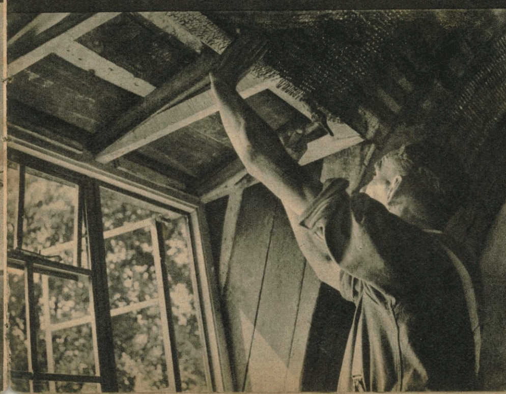
A bay window is being made. The construction is partly of wire mesh, which the Guardsman seen here is "peeling over."
