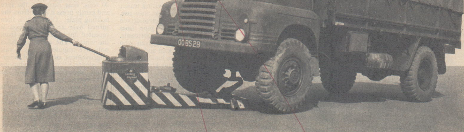
"Look, one hand!" A WRAC corporal demonstrates how a three-ton lorry can be pulled along by a mobile electric jack.
