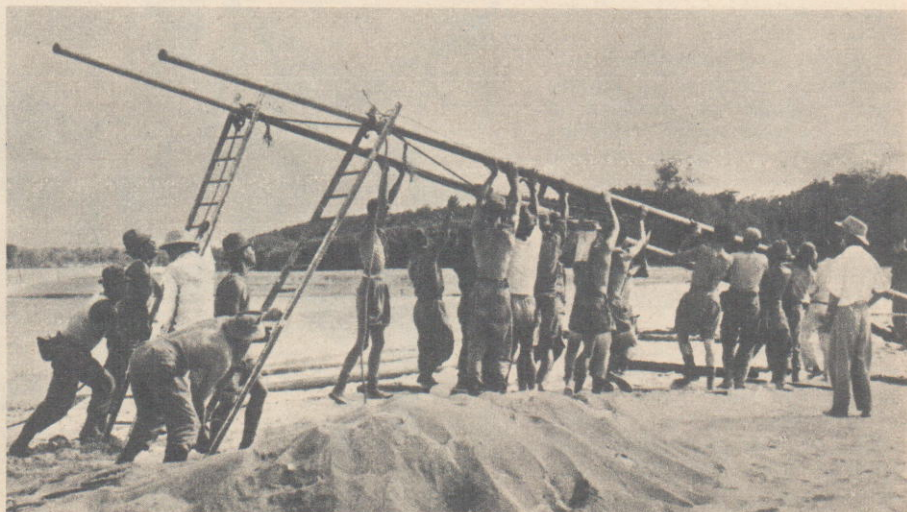
Troops of three nations hoist one of the "H" poles into place to take the line across a river.
