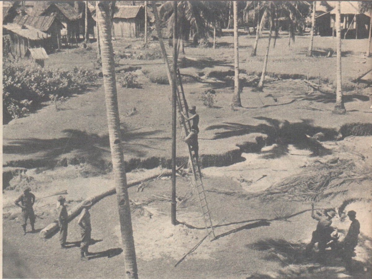
On a coconut palm plantation in Pontian, British and Australian soldiers erect one of the 520 poles. It was not all such easy going. For ten miles, the Signalmen had to fight through swamp and jungle.
