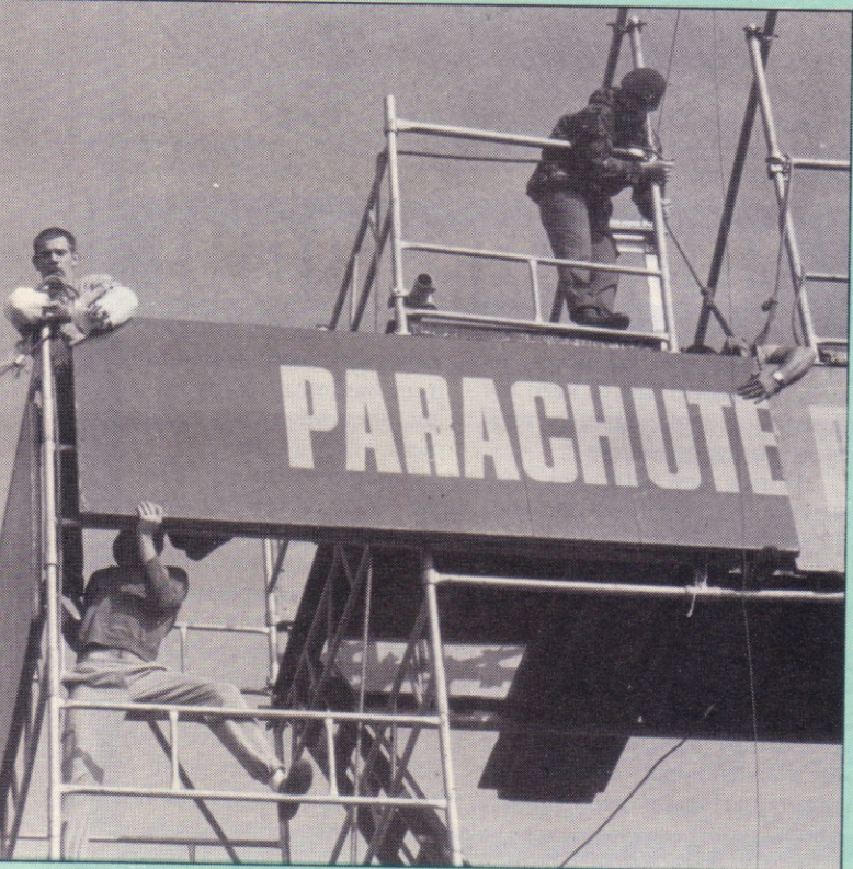
Pte 'Boy' Gray hammers in one of the tower anchor bars.
