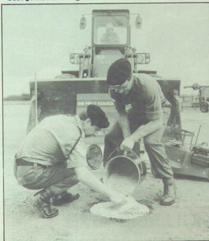
Cpls Jim Taylor and Fred Crudge repairing holes in an airfield.
